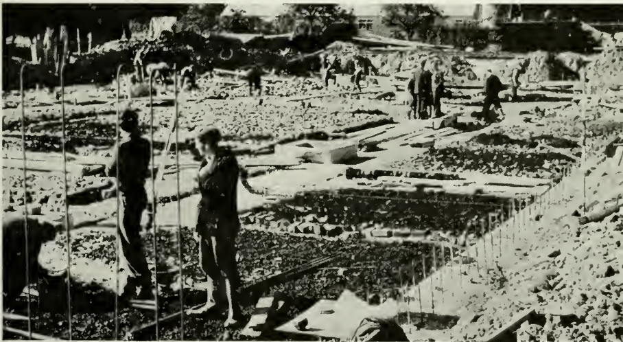
The installation of the footings
